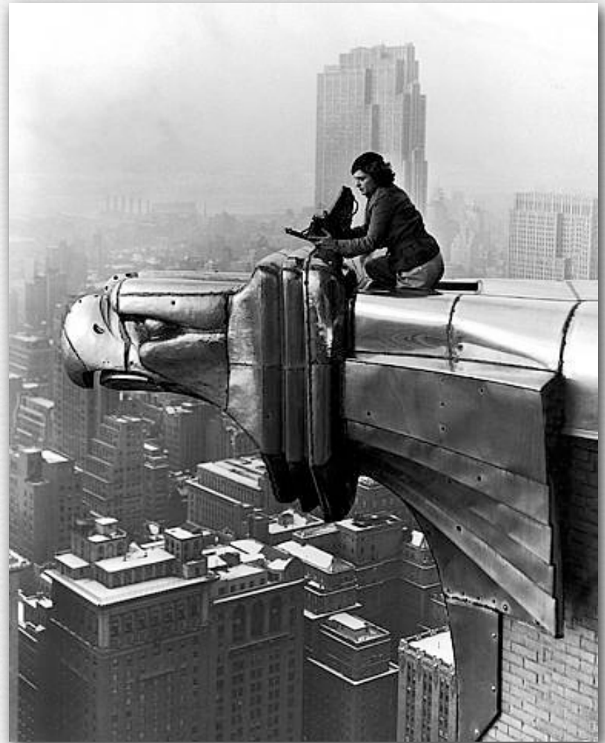
Margaret Bourke-White atop the Chrysler Building
