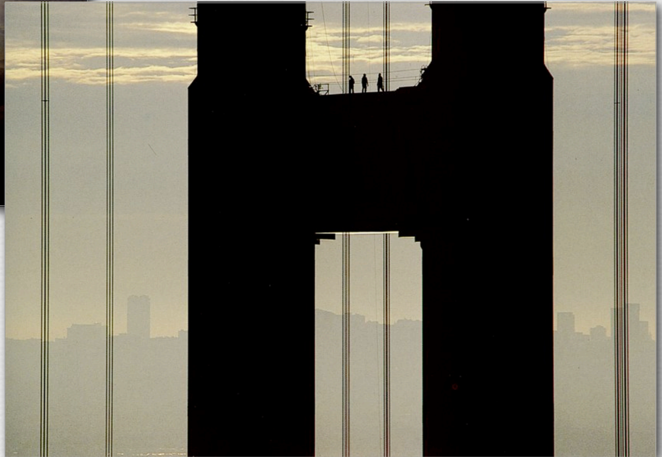
Bryan Peterson, Golden Gate Bridge
