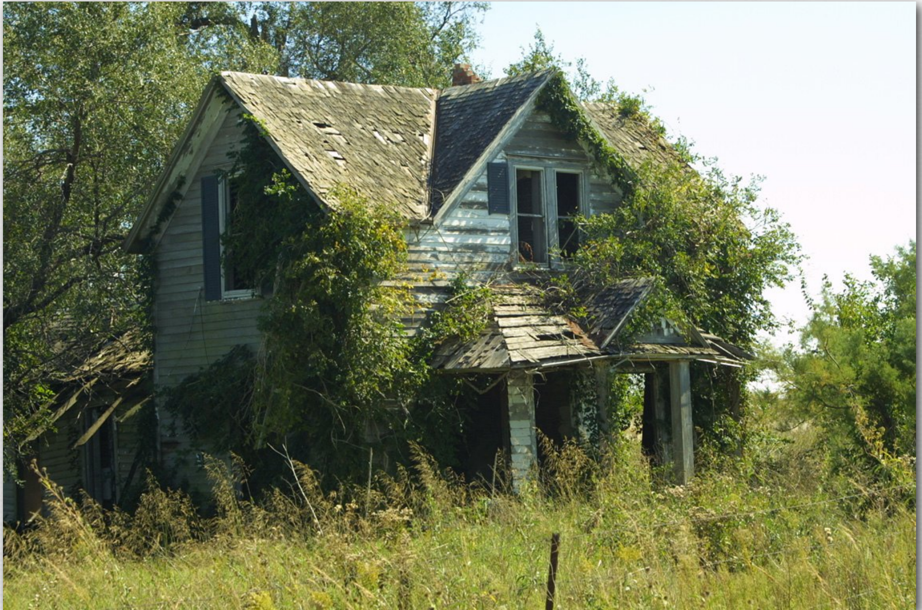
Abandoned farmhouse, Kansas
