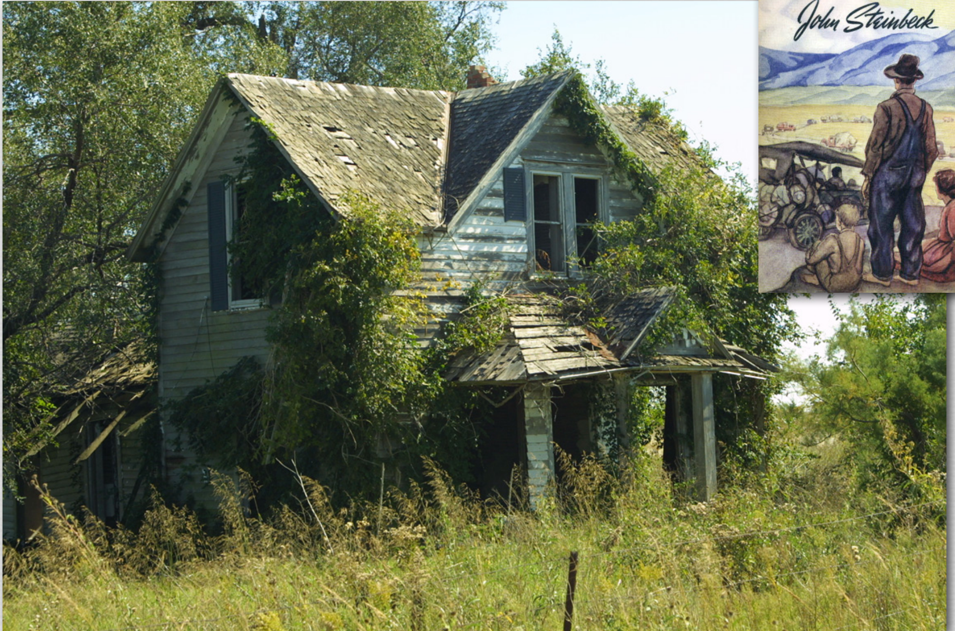
Abandoned farmhouse, Kansas
